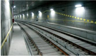
Ballastless track now includes also embedded block track and embedded rail track as parallel categories to direct-fixation track.
