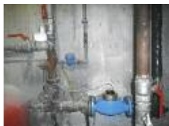
Smart Meter installation
