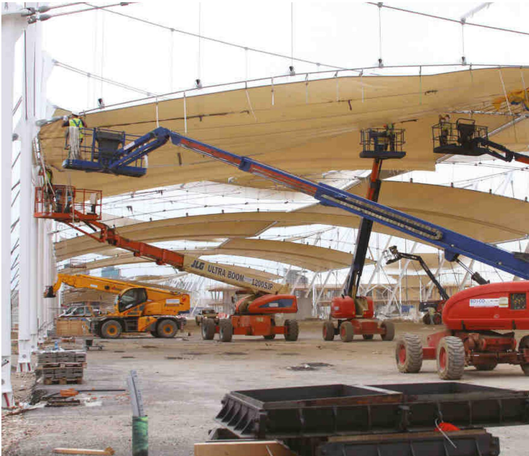
*two cables, bearing and stabiliser, had an oppositely configured curvature and were pre stressed by means of a force-field of vertically self-balancing traction; the pre-stressing was applied by hydraulic jacks acting on the adjustable cable-heads positioned at the end of the stabilising cable;*
