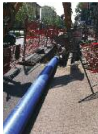
Slip Lining DN 400
