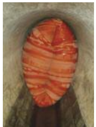
Cured In Place Pipe
