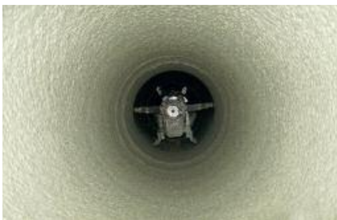
Cement Mortar Lining DN 1000
